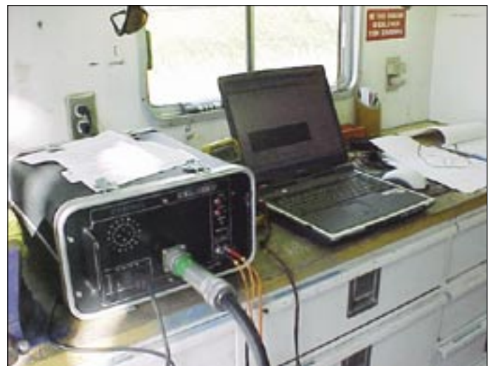
Figure 2 — Installation of the recloser analyzer, GEN-3/12, on a Cooper recloser with F3A control at a Hydro-Québec substation
