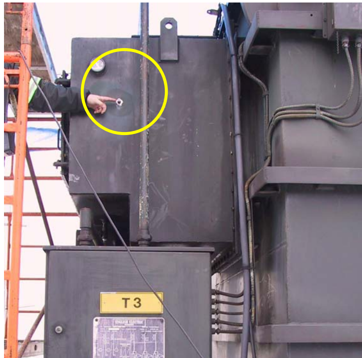
Figure I.7: Internal setup of the OLTP conduit for a particular choice regarding the location of the probe.
