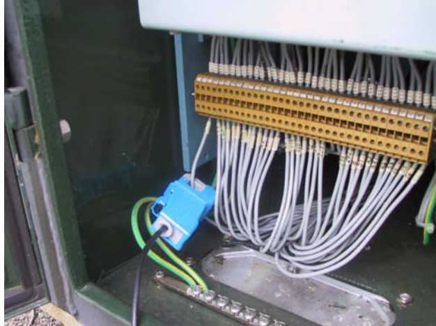
Figure 4 : The clamp can be installed on a wire identified by the terminal block or near the motor as long as the wire is marked for subsequent measurements.
