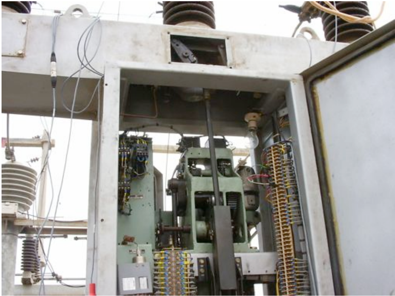
Upper part of mechanism in open position.
