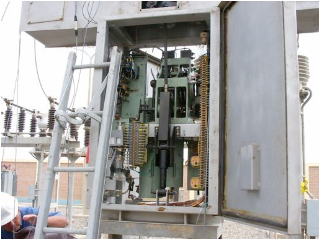
Lower part of the linear displacement mechanism on a candle-type circuit breaker.
