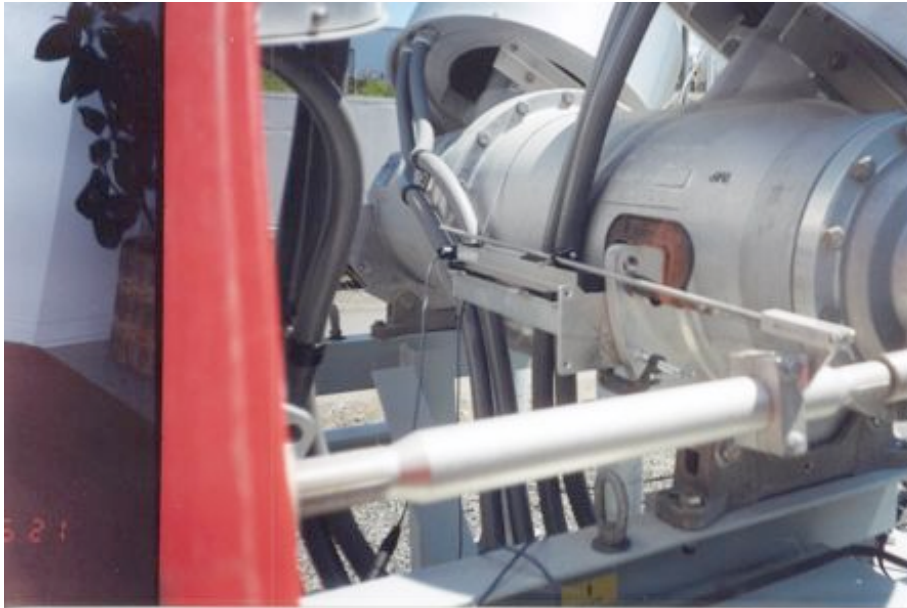
Linear transducer adapted to ABB breaker.
