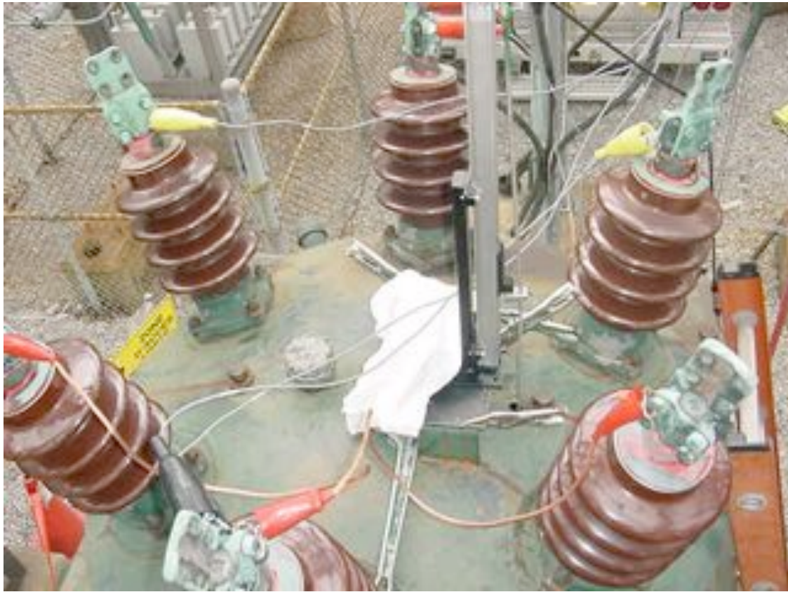
Linear transducer and base attached to the breaker.
