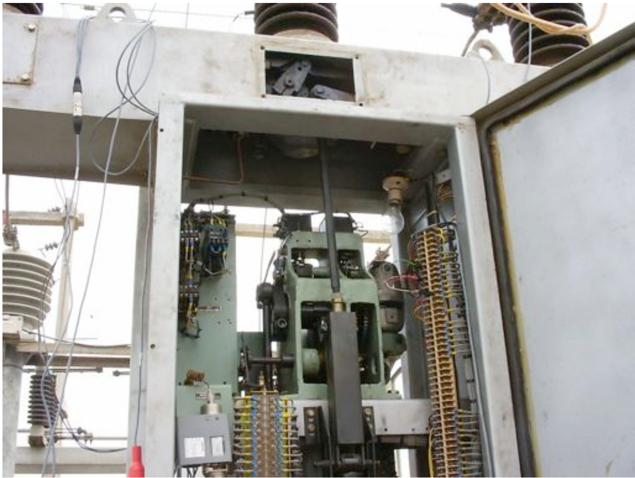
Upper part of mechanism in closed position.
