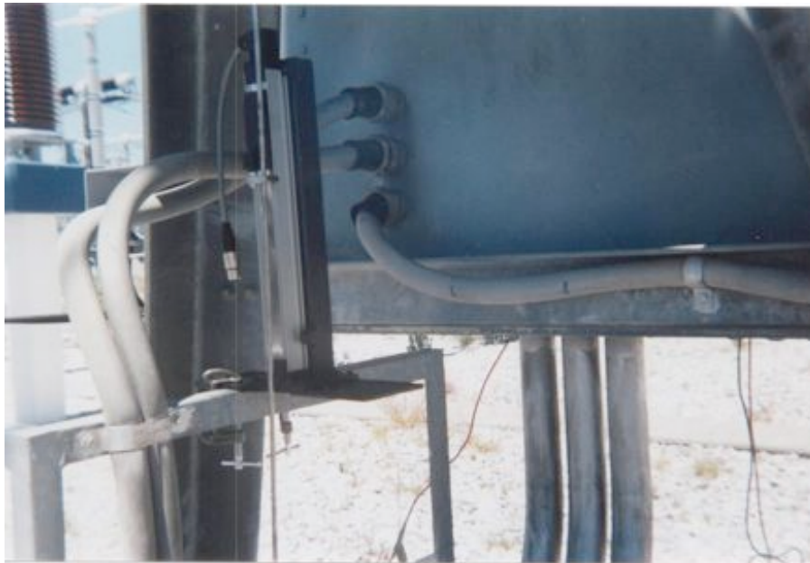
Linear transducer mounted on 6-contact SF6 breaker.
