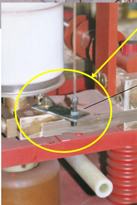
The displacement of this breaker is very small (less than 1/2 inch). The rod was attached to the breaker with a simple steel plate.
