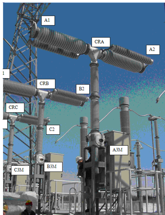
Figure 28 Accelerometer location
