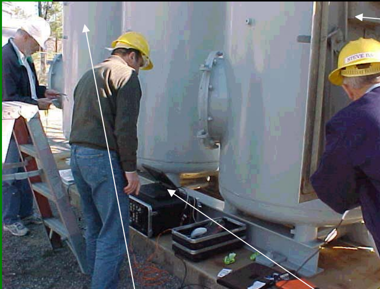
Breaker with 3 separate tanks
