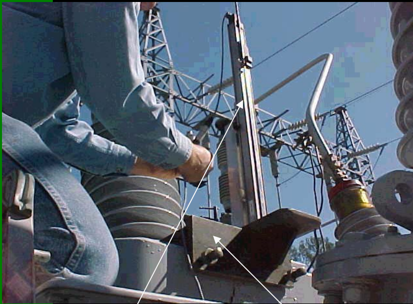
Linear travel transducer
