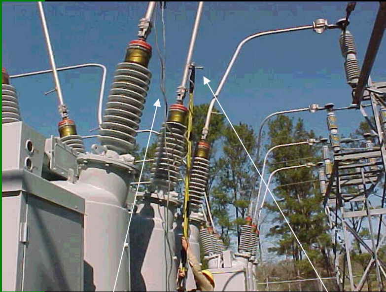
Grounding of the breaker
